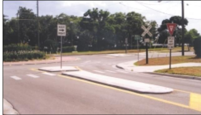
All except mini-roundabouts have raised splitter islands. These are designed to separate traffic moving in opposite directions, deflect entering traffic, and to provide opportunities for pedestrians to cross in two stages. Mini-roundabouts may have splitter islands defined only by pavement markings. *Tavares, FL*
